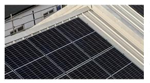
Last month 360m<sup>2</sup> of solar PV panels were installed on the roofing of all three of CP Cases' factory units. This includes maximum coverage on Units 6 and 11, and a strip of panels on Unit 10. Skylights on this roof made it unsuitable for complete coverage.
