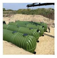
Roto Group congratulates Roto Hungary on their new project which has now been completed. A new injection moulding plant in Székesfehérvár, required a 230m<sup>3</sup> combined firewater and stormwater storage system. This 230m<sup>3</sup> system consists of three Roterra 2450, 60m<sup>3</sup> tanks and one 50m<sup>3</sup> tank.
