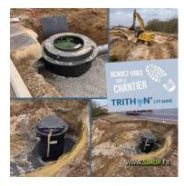
TRITHON hydrodynamic separators, produced by SIMOP, have been installed to protect the natural surroundings of an industrial site that deposits small amounts of pollution on the ground (micro-plastics, industrial plastic granules (IPG), hydrocarbons, tyre particles, etc.).
